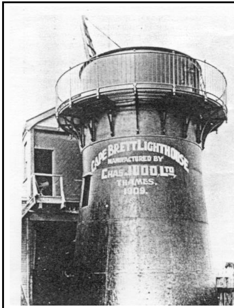
Figure 15 - The cast iron tower for Cape Brett constructed on the Judd foundry in Thames.
