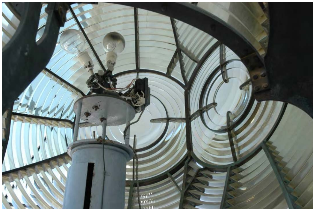
Figure 25 – The current lamp fixture.
