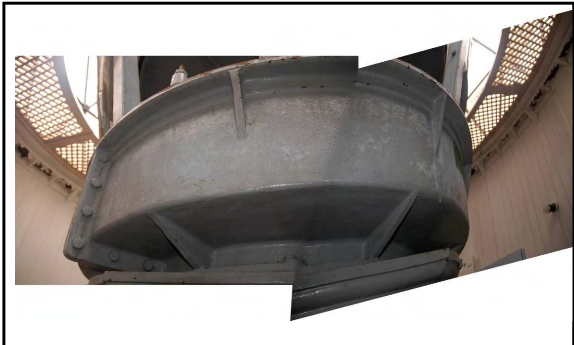
Figure 30 –The mercury bath.
