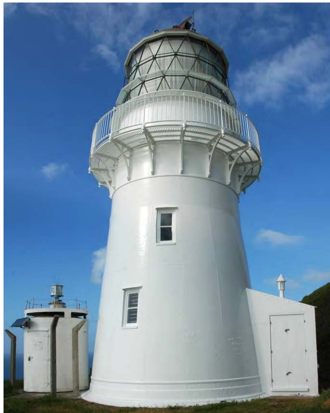
Figure 35 – The made-over lighthouse, straight after the painters had finished.
