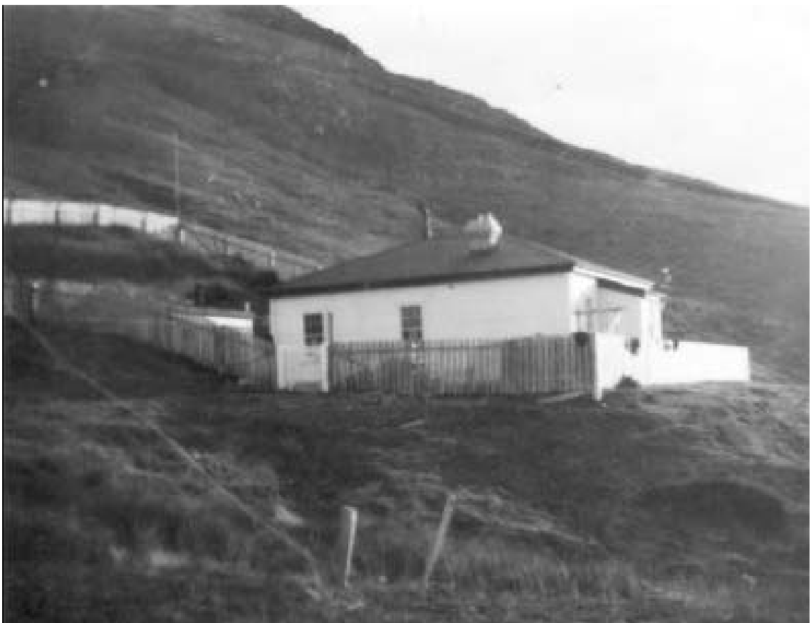
Figure 57 – The third house from the east.
