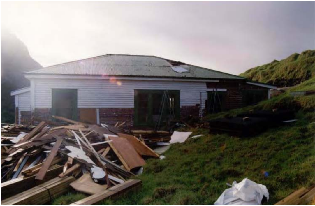
Figure 54 – The hut in the process of being refurbished, 1996.
