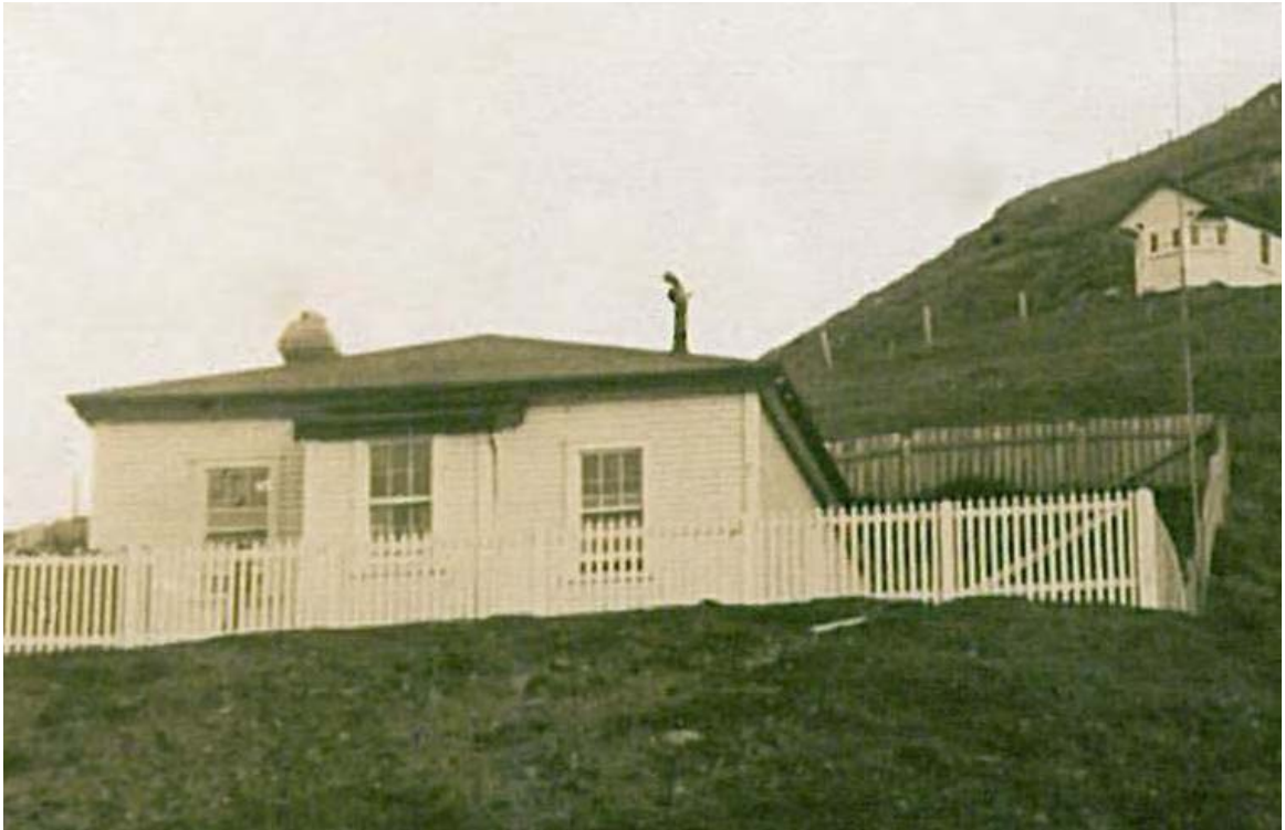
Figure 56 – The front view of the third house with the signal hut in background.
