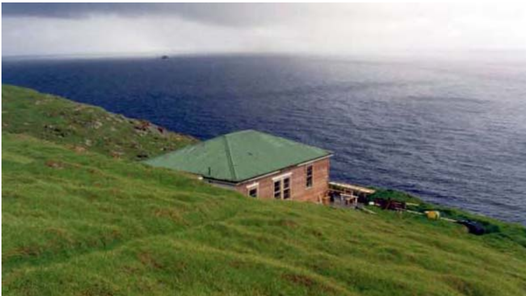
Figure 55 – The outside of the second house in the process of being painted, 1996.
