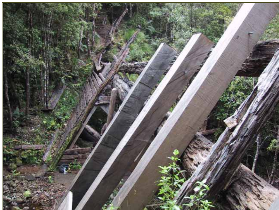
Christmas Creek dam restoration 1998. Photo: N.Ritchie
