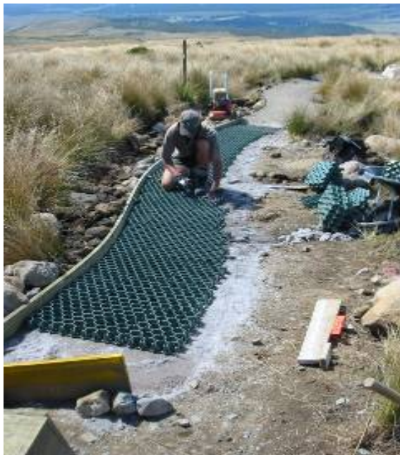
Figure 56 – Geocells are easily cut to any shape to fit the “flow” of the track
