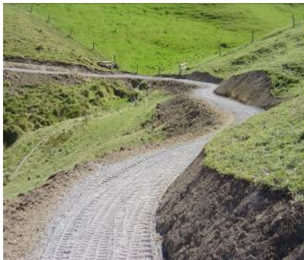
Figure 28 - This is a good example of a full bench cut
