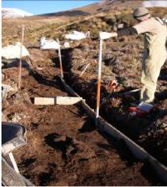
Figure 55 – Timber edging is bent to ensure the track flows and reflects the landscape
