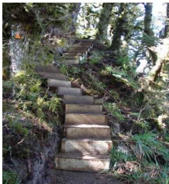
Figure 80 – Aesthetically boxed steps are a good option for large rises. As you are able to produce a segmented curve they are more visually acceptable within the landscape
