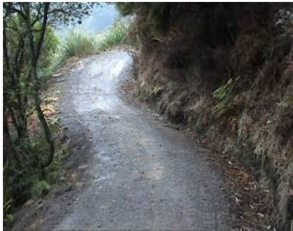
Figure 15 - This very subtle grade dip produces a very short point to point track surface
