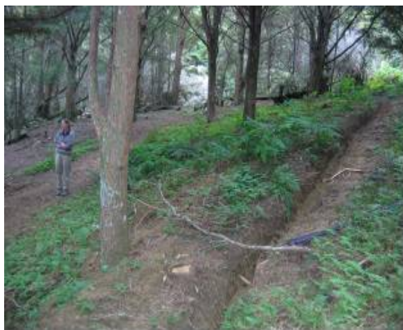
Figure 37 - This catch drain is not visible from the walking track and collects water from the sideslope before it reaches the track
