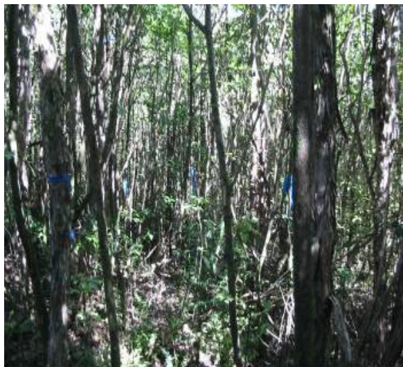
Figure 21 - Take the time and effort to mark your track well. It will help to avoid poor alignment by those constructing the track
