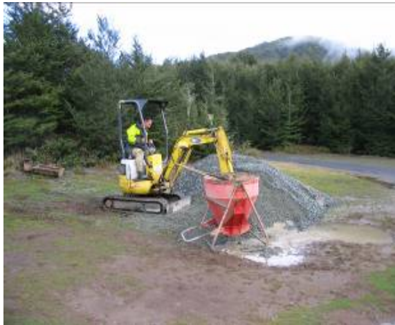
Figure 68 – Loading with the correct size digger makes an efficient operation.
