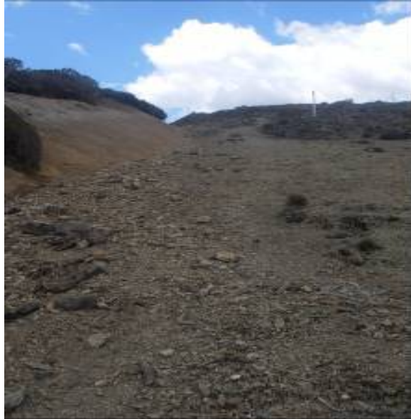
Figure 27 - Not all tracks require formation work. This tramping track has significant lengths of unbenched track in excellent condition
