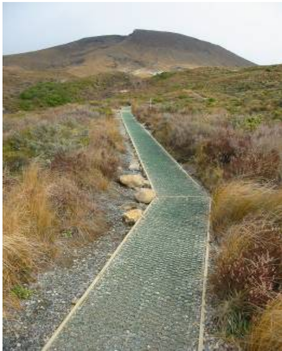
Figure 60 – While this section of track could be significantly improved aesthetically, it demonstrates that the geocells are effective in holding material. The gradient on this section of track is 13°
