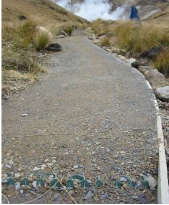
Figure 59 – Completed section of track showing geocells and compacted walking surface.
