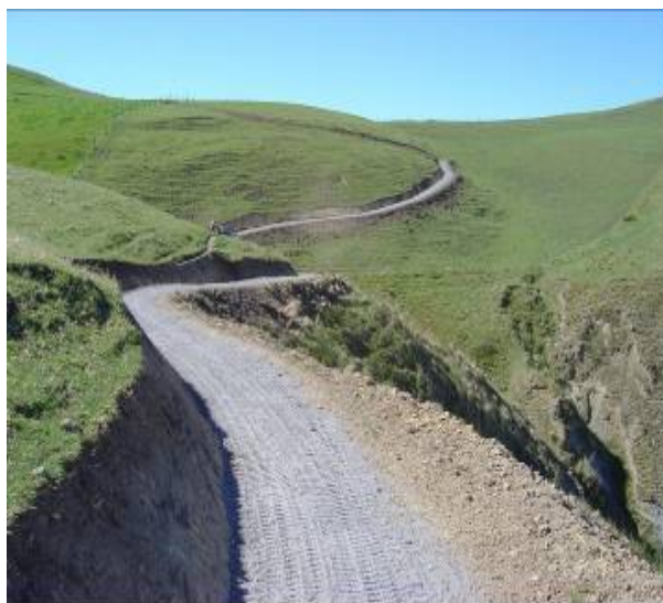
Figure 30 - The batter on this track is formed at an angle close to the sideslope angle giving the track a “softer” visual appearance
