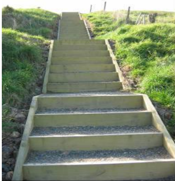
Figure 70 - Steps introduce straight lines into the natural landscape, where there are few perfectly straight lines, and look out of place. When selecting the location of steps look at the site from above and below
