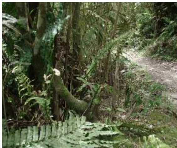
Figure 97 - For the same effort this “hanger” could have been cut at ground level giving a considerably neater appearance to the finished track
