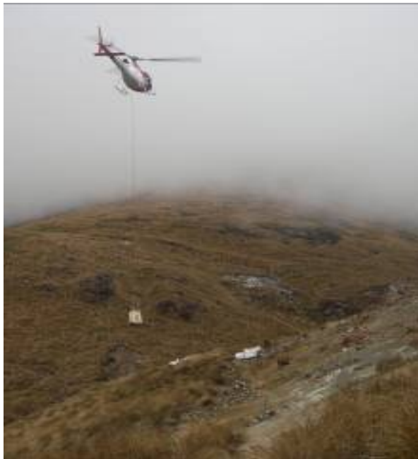
Figure 65 – Knowing the volume of material in each fadge and the distance this will cover on the track allows fadges to be placed in the correct location
