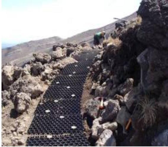
Figure 61 – Edging is not always necessary and these geocells will be covered with an acceptable walking surface
