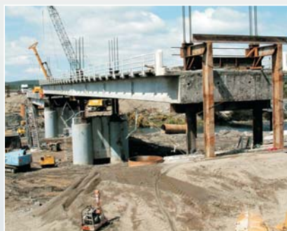
State Highway 49 bridge being raised and strengthened.
