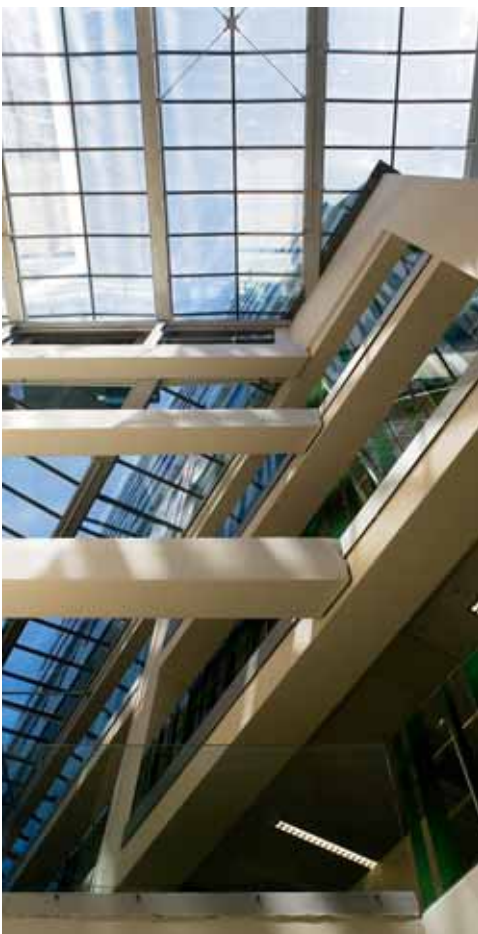
Above: Along with natural light, the atrium also provides natural ventilation as fresh air from the rooftop is circulated through the atrium and back up to the roof via the double facade.
