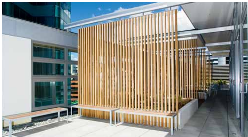
Right: Running along the Manners St perimeter of the building and flanking the cafe, the double facade is used to flush used air out of the building at night.
