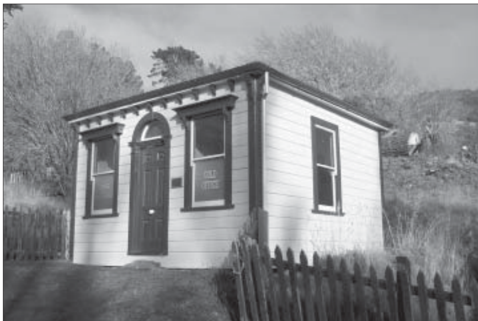
Figure 18. Gold Office as viewed from the main street.
