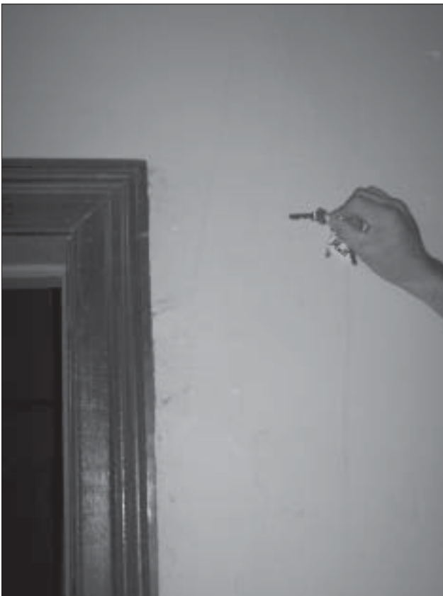
Figure 33. Re-plastering work adjacent to door to SWC office.
