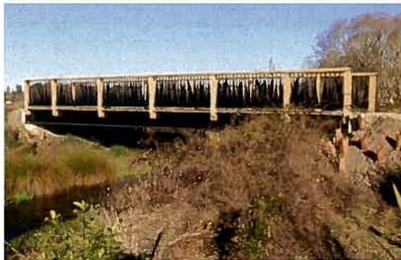
Bridge over Otukaikino Stream (Photo: B Rule)
