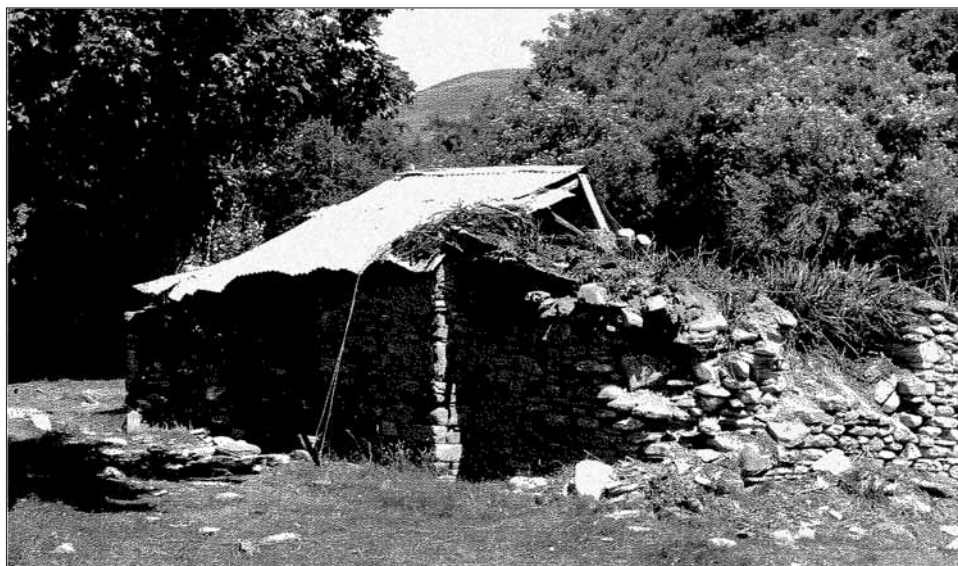
Figure 4. The Bakehouse (from the northwest) in the late 1970s, showing the front (north) elevation on the left. The large stone filling a hole at the near end of the front wall may be obscuring an oven entrance. Note the shelf-like stone below the hole. 2 Photo: L&S records from DOC files.
