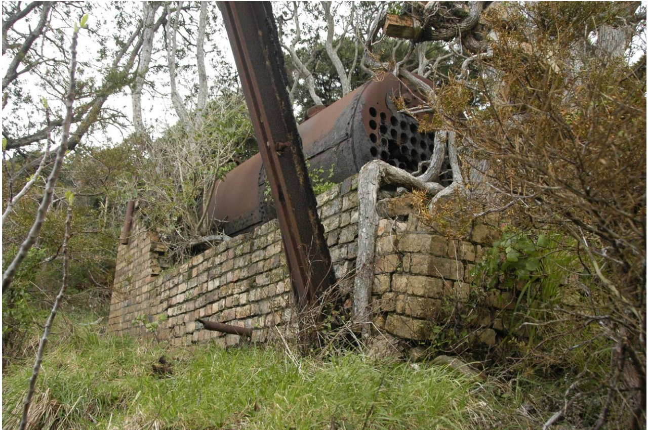
Figure 4: The steel boiler at Whangamumu that powered factory operations, (A. Blanshard 2009).
