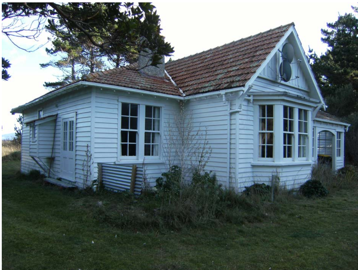
Figure 1: Cottage/pilot house No. 1 photo (July 2015)
