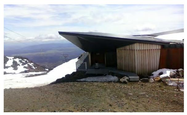
Image 7 - Photo showing the east side of the Knoll Ridge Café, and an example of the suite of materials being used on the Whakapapa Ski Area buildings – dark iron sand colour steel, weathered timber cladding, corten steel, tinted windows. Photo taken October 2015.
