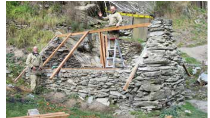
Before A hut during restoration.
