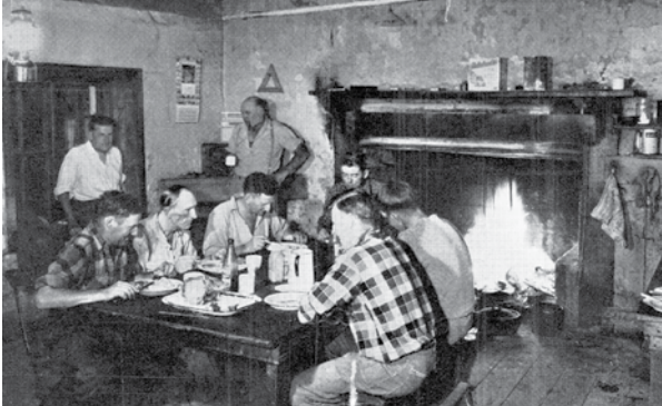
On the day of the muster breakfast at the Tynedale homestead was at 3 am. The sod-walled building is nearly 100 years old.
