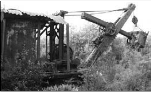
Figure 7. The Haupiri steam shovel, West Coast. Photo: Jim Staton, Greymouth Area Office, DOC.
