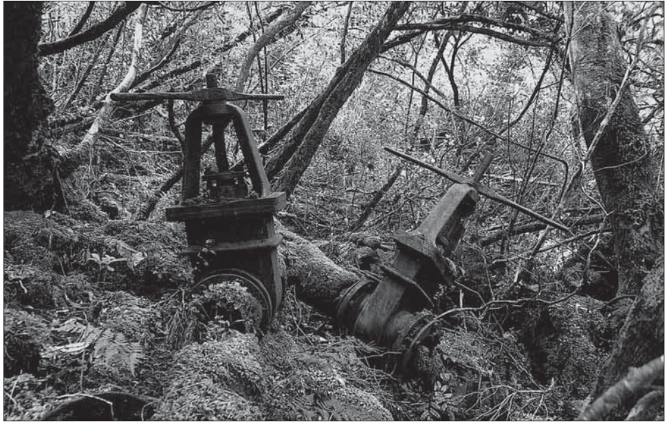
Figure 16. Two screw (gate) valves at the end of the main pipeline, Site D49/41. Photo: P. Petchey.
