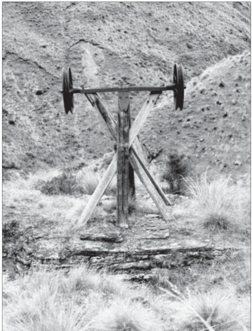
An aerial cableway pylon, Homeward Bound cableway (see Section 7.9.1). Photograph: P. Petchey.
