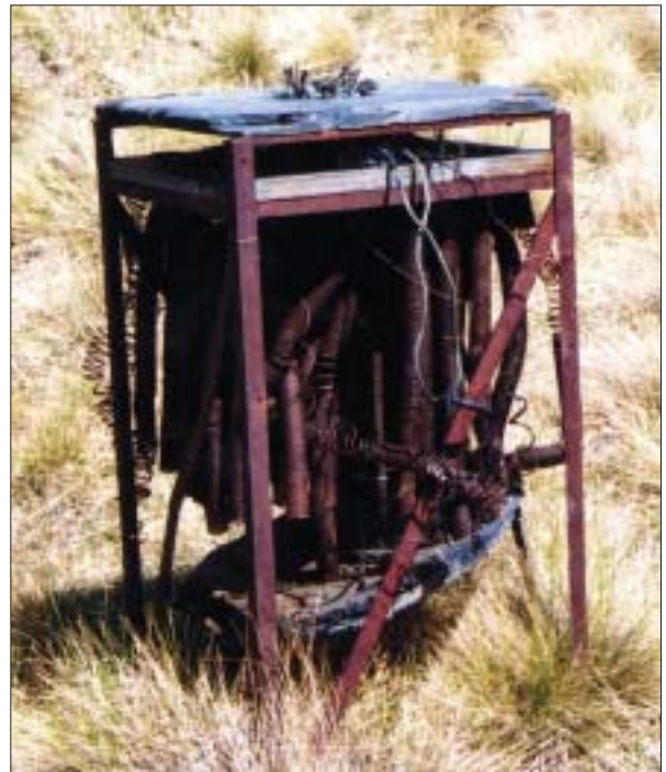
Figure 42. Variable resistance controller for the Premier Mine generator. Photo: P. Petchey.
