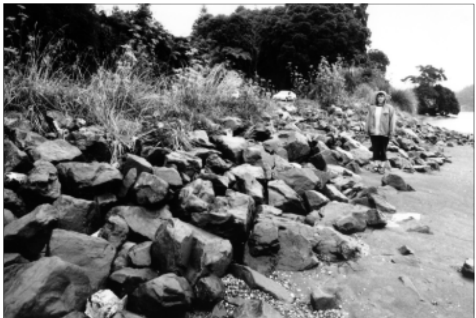
Figure 8. Rip-rap sea wall protecting areas of the site of Tokitoki, Ōhiwa Harbour.
