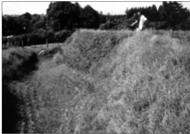
Figure 11. Partly mowed grass cover on the ditch and bank of a redoubt at Pirongia, Waipa district, Waikato. The banks are stable and the grass is probably weed-eaten once or twice a year. The base of the ditch is mown by a small ride-on mower. The pattern of varying grass heights in the ditch tends to obscure the profile of the ditch and bank but is satisfactory.
