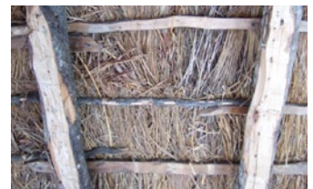
Beech rafters and tussock thatching.
