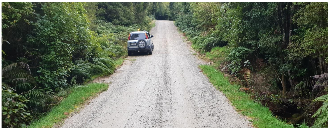
Figure 38. Low stature forest typical of section E, with adequate road width to form a wider road surface without having to alter the drainage markedly. Most of the vegetation requiring removal would be exotic species plus kiokio and small shrubs and tree ferns.
