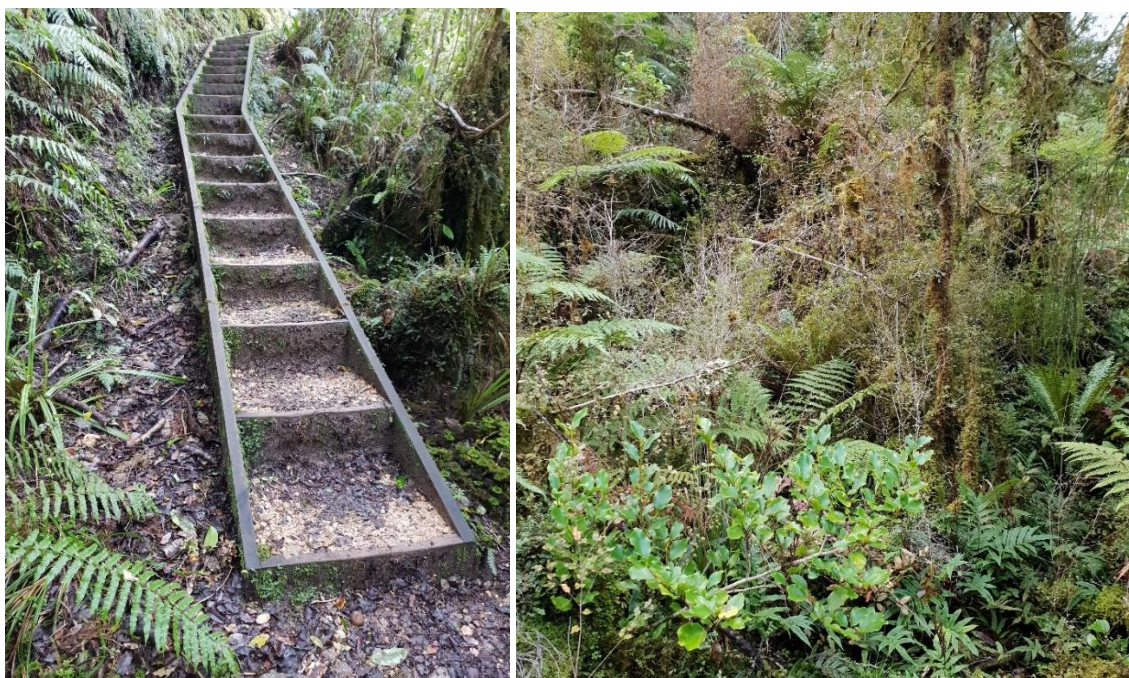
Figure 15. Steps lead up from the existing terrace and across the limestone bluff on which the elevated walkway is proposed. The flight of steps has an overall gradient of about 22° but are only 600mm wide compared with the existing track surface of more than a metre.
