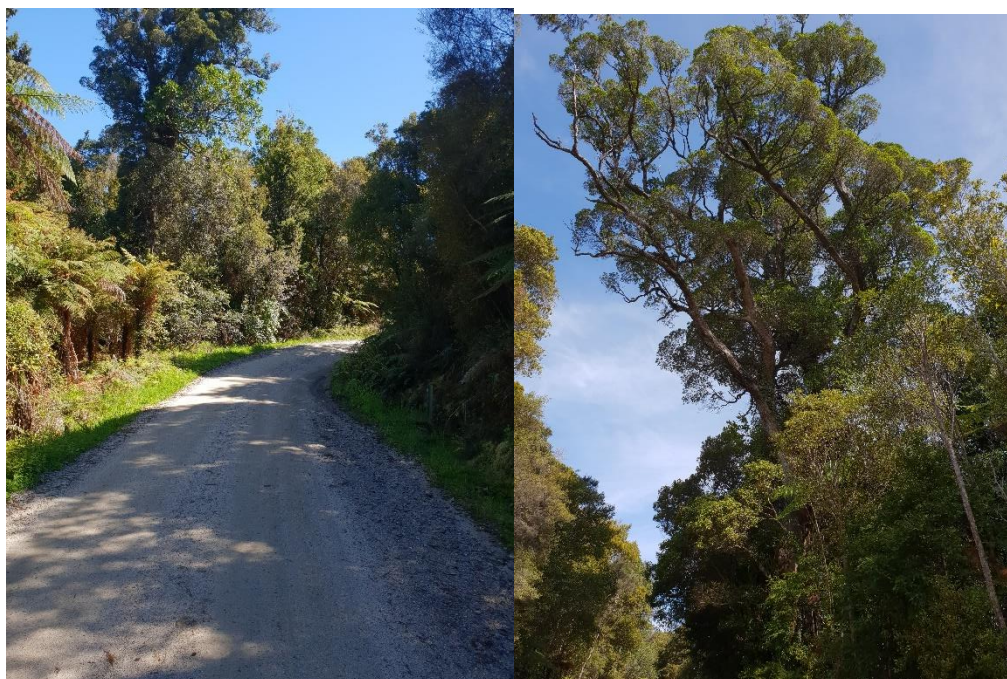
Figure 31. Typical vegetation along broad sweeping curves and gentle gradient of section A. There is generally enough room to easily accommodate a wider carriageway without affecting a significant amount of indigenous vegetation.
