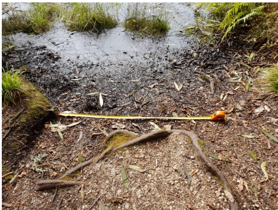
Figure 46 showing width of proposed structure (1.2m), as well as devegetated area on lake edge with exposed tree roots.
