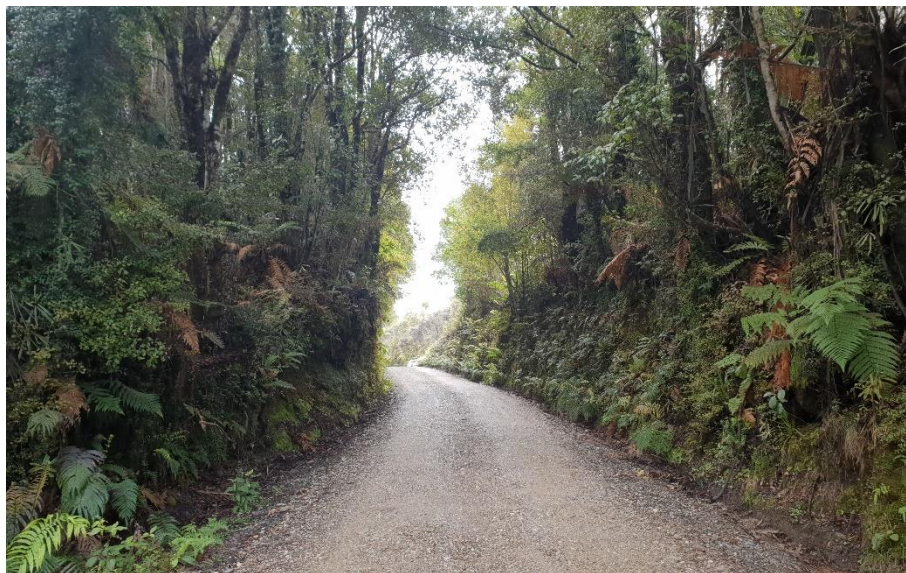
Figure 36. Abbotsford cutting. Clearance of kiokio and some small trees, including red beech, kāmahi and northern rata would be required on this short section.
