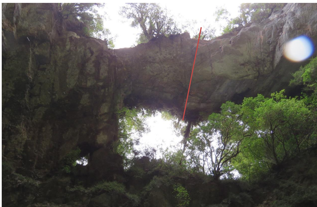
Figure 13 showing zone of weakness that presents a rock-fall hazard to track-users. The current proposal would allow visitors to view the arch without exposing them to a direct risk from arch collapse.
