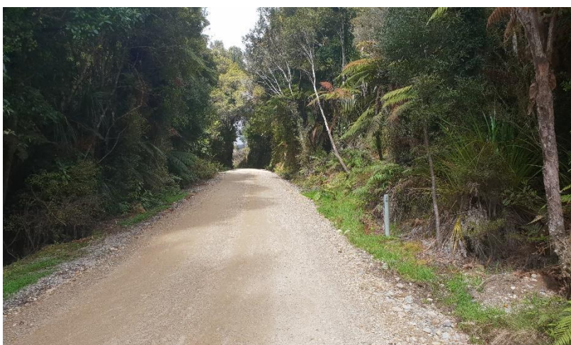
Figure 32. The climb up to the top of the rise on section B. the gradient is about 8° and while there is generally a reasonable amount of room to extend the road width, some native trees will need to be felled to accommodate a 6m carriageway.
