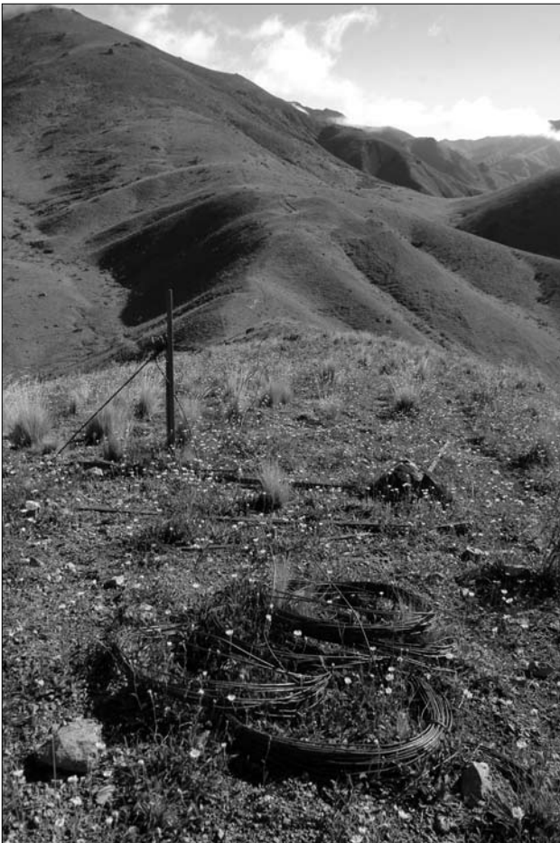
Figure 14. Dismantled rabbit-proof fence, showing detail of the strainer post and recovered rolls of wire at Saxton Pass, Molesworth. Photo courtesy of Kevin L. Jones, DOC.
