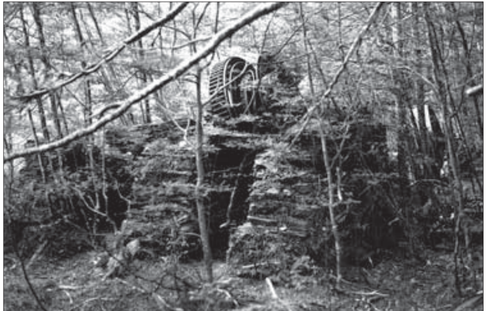
Figure 14. New Main Shaft, 1996. Cossons & Black winding drum and foundations.
