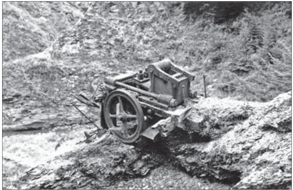
Figure 22. Kincaid & McQueen rockcrusher. Note decayed support timbers. Photo: P. Petchey.
