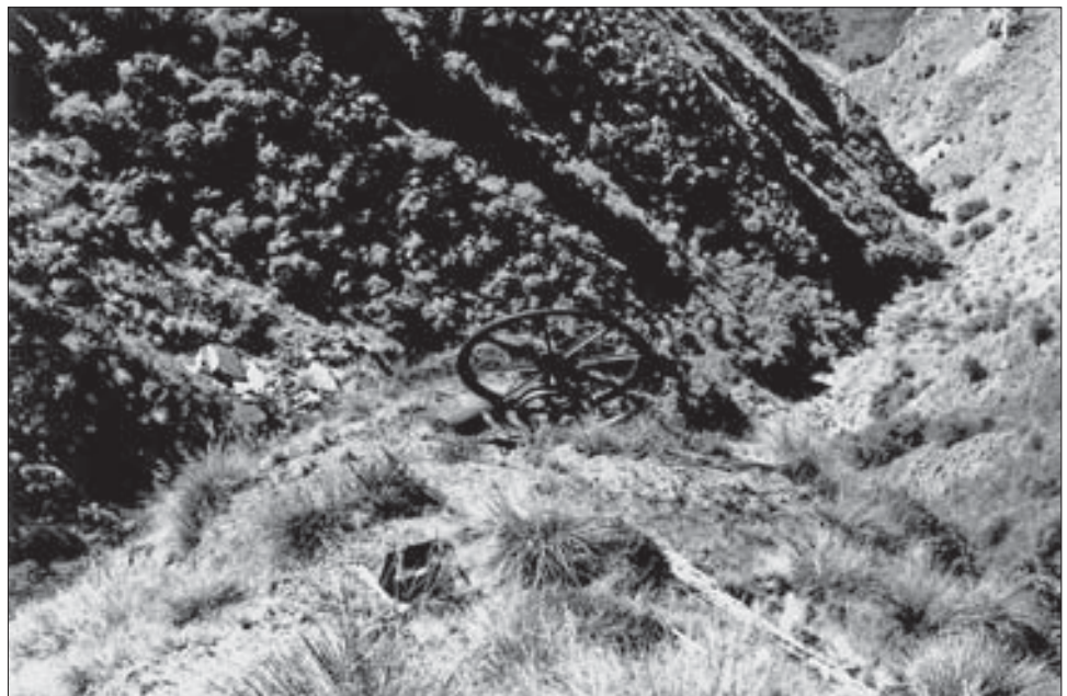
Figure 11. Aerial cableway terminus wheel on British-American Spur, 1996. Photo: P. Petchey.
