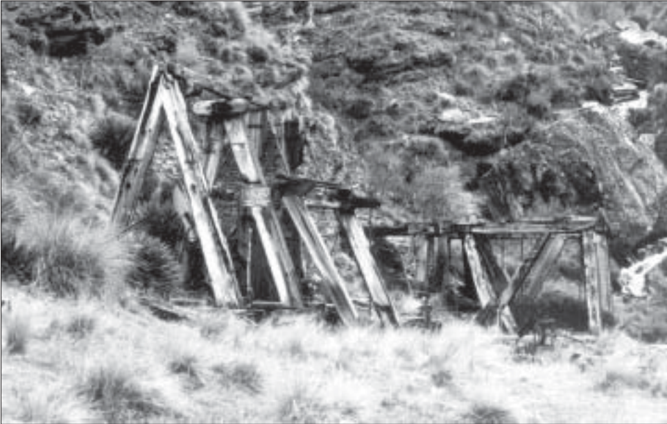
Figure 40. Maryborough/ Premier Battery stand and water wheel race supporting structure from the southeast. Photo: K. Jones, Department of Conservation, Wellington.
