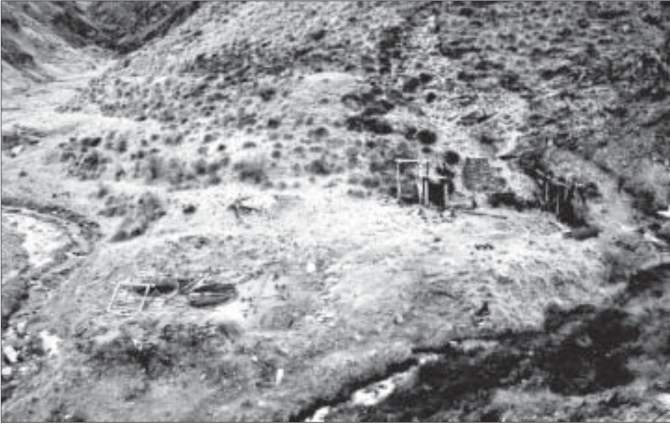
Figure 39. Maryborough/ Premier Battery site from the northeast. On the left are the cyanide tanks, and to the right the remains of the stamper frames and the water wheel frame. The Rich Burn runs in from the right, and Sawyers Creek is on the left. Photo: P. Petchey.
