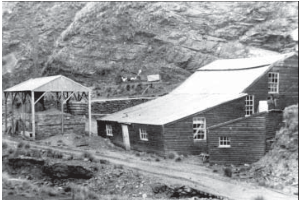
Figure 25. Tipperary Battery c. 1900. The furnace can be seen under the open-sided shelter to the left of the building housing the battery. Photo: Lakes District Museum, Arrowsmith.
