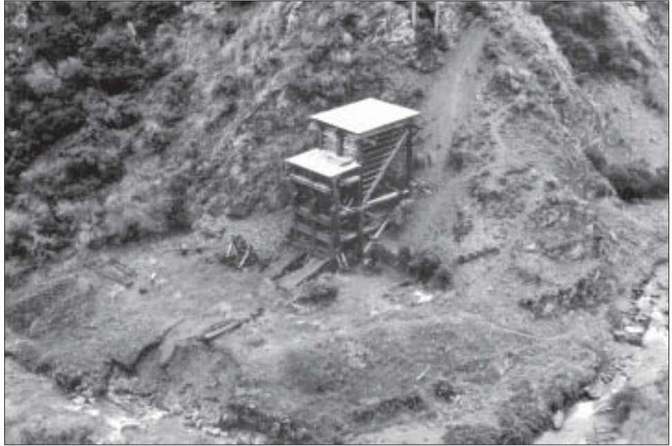
Figure 19. The remains of the third Homeward Bound Battery (ex OPQ). The roof on the structure is a recent addition to slow down the deterioration of the timbers. The berdan is in its correct position, but the camshaft and Wilfley table have been dismantled. Photo: P. Petchey.
