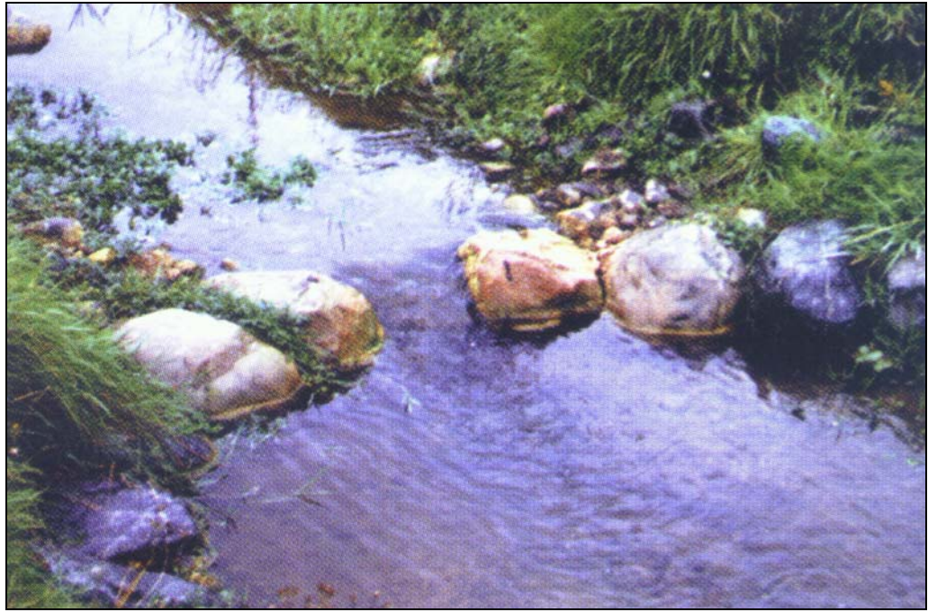
Plate 9. V-notch weir constructed from rocks. Note that each rock leans on the one down stream to ensure the stability of the structure. The central rock (submerged) is the lowest so as to create a notch in mid channel.
