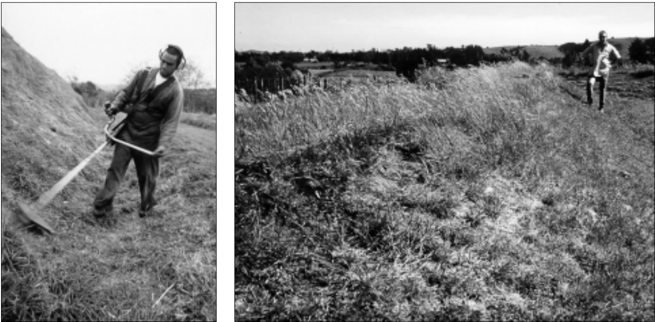
Figure 32. Good and bad in grass cover management. (A, left) Banks should be cut by a weed-eater; (B, right) ride-on mowers often create scalping where there is a rise in the ground surface.
