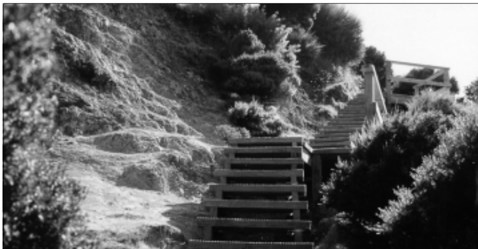
Figure 31. On Motuarohia, Bay of Islands, steps and railing to an accepted engineering standard on a severely eroded track to a viewpoint on the exposed platform of a pā.
